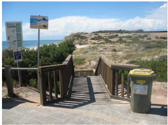
Formalised access path with Hooded Plover signage. Photo Grainne Maguire.
